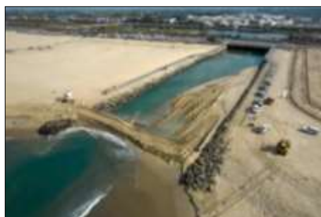
A temporary sand berm sits at the inlet to the Talbert Marsh to prevent more oil from entering the wetland in Huntington Beach, CA on October 4, 2021
