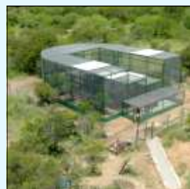
Later, the U-shaped aviary was completed
